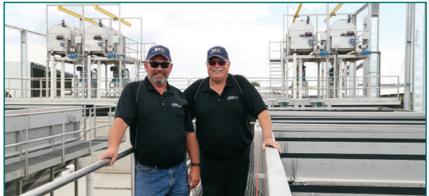
Kerry Doyle (right), founder and CEO of Trident Processes LLC, and R.C. Ludke (left), President, inspecting a site after the installation of a Trident nutrient recovery system.
